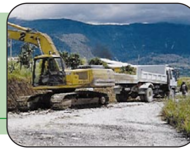
Road construction at Palam
